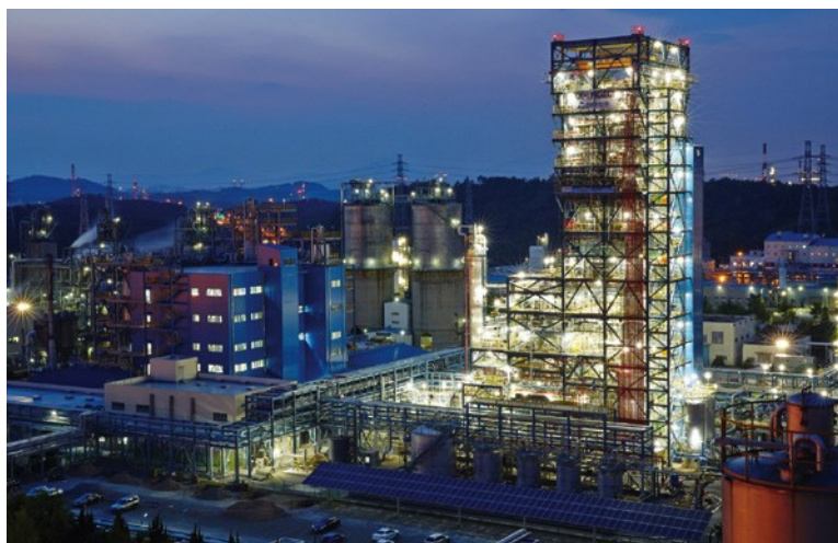
Above: Hyosung's 50,000tpa commercial-scale PK facility in South Korea started up in July last year
